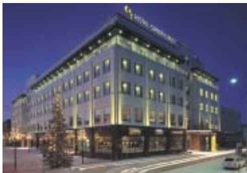
Hotel Santa Claus - Rovaniemi (Finland) Heating & cooling installation with ASV valves
