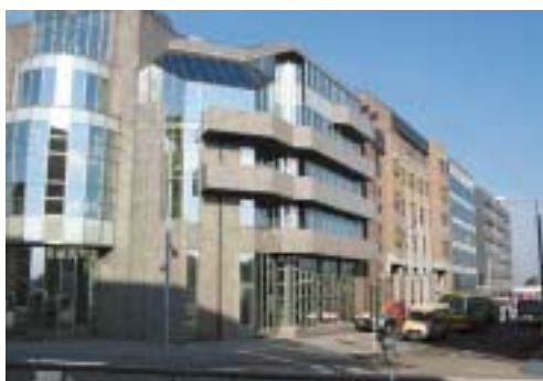
KBC-Bank - Leuven (Belgium) Chilled air system installation
