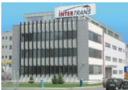
Intertrans - Ljubljana (Slovenia) Cooling system installation with ASV-Q valves
