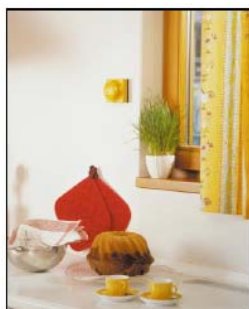
Photo 2 A sensor installed at a distance, ideal for inaccessible radiators
